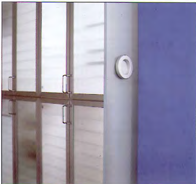
Figure 4: The walls have through and through cupboards and shelves
