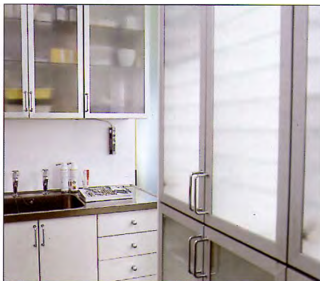
Figure 3: The sterilising rooms all feature one-piece stainless steel customised worktops
